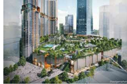
Mix Use Development - Malaysia Lendlease
