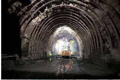
Tunnel Construction - Lyon Turin Eiffage / Spie Batignolles
